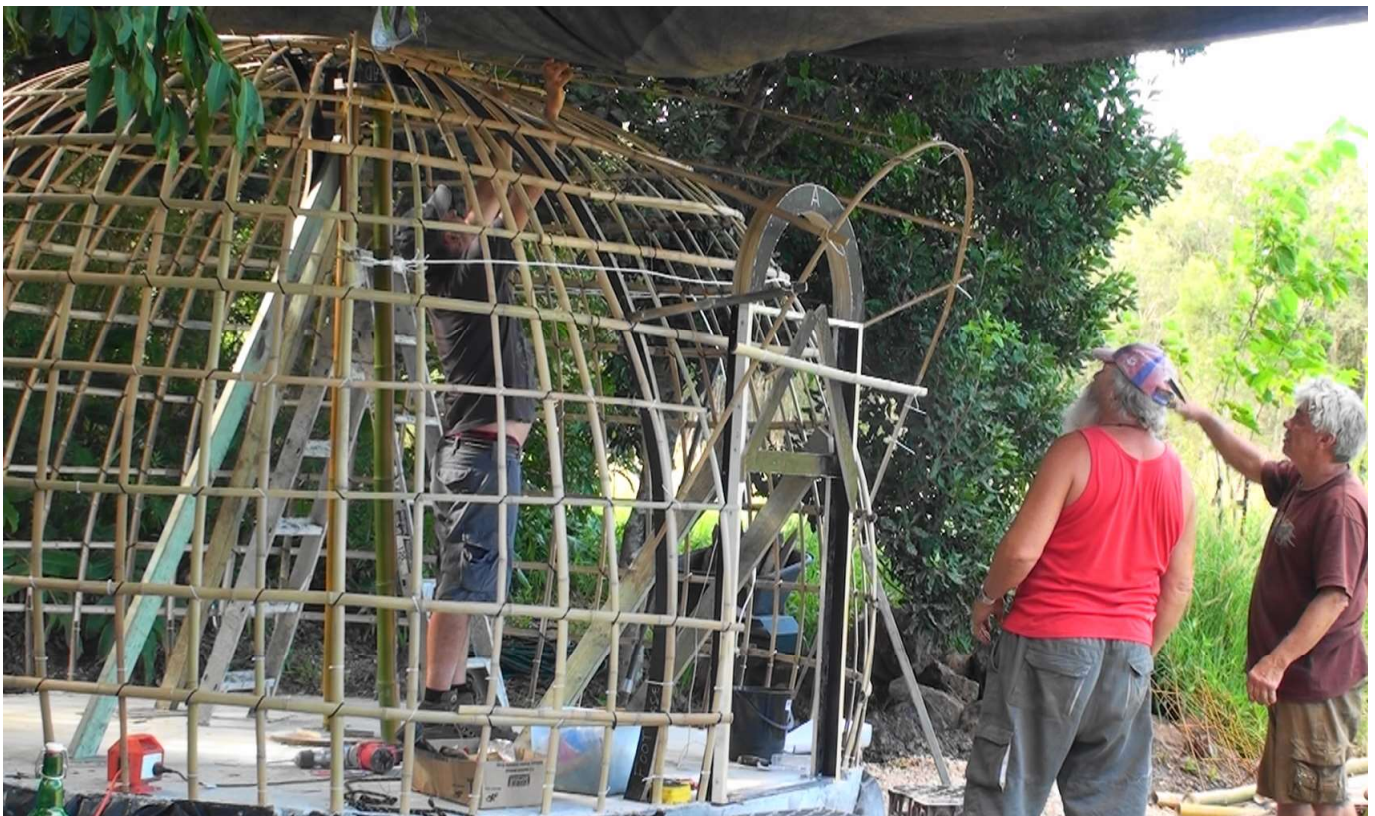
Creating the profile shapes of the hood over the doorway.
