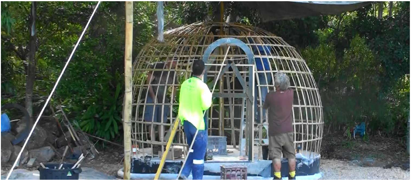
Creating the profile shapes of the hood over the doorway.
