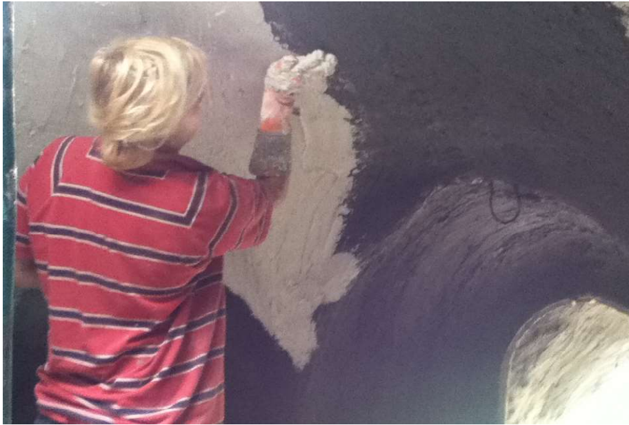
The Difference after the First Coat of White Plaster
