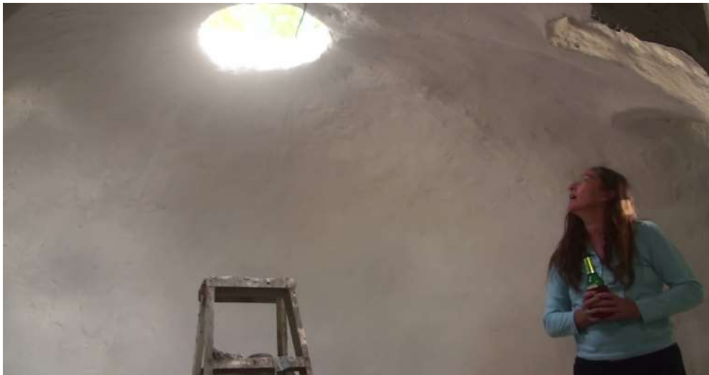
The Difference after the First Coat of White Plaster
