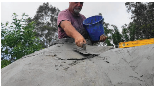
A thin sheet of plastic around the hob helps smooth it off, keep it circular and allow for taking a level
