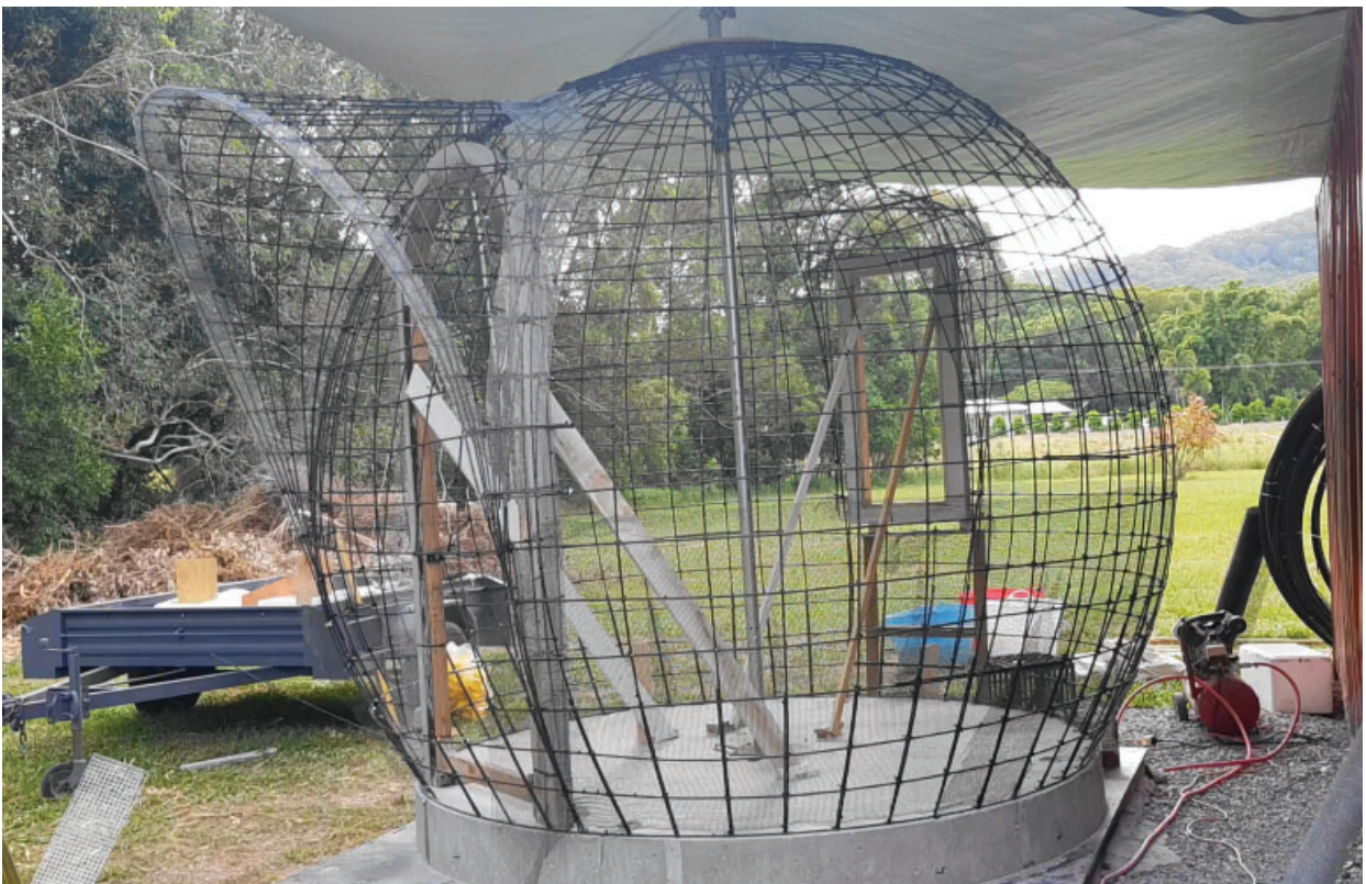
A framed up dome cage WITH the window and door hoods fabricated
