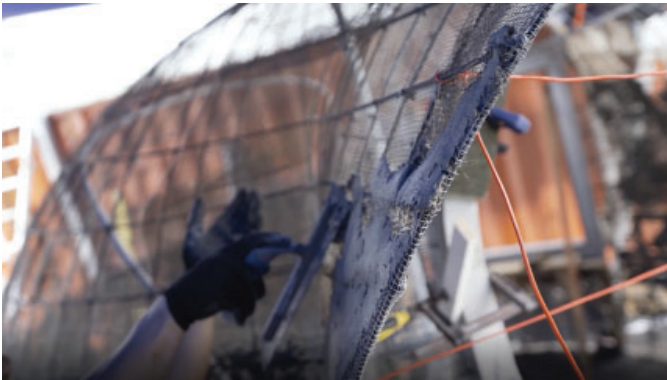
Gently applying render to the hoods by hand trowel
