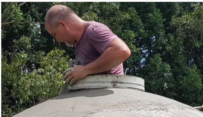
A thin sheet of plastic around the hob helps smooth it off, keep it circular and allow for taking a level
