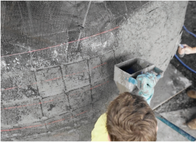
Gently applying render to the hoods by hand trowel
