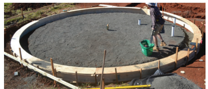
Formwork fixed - sand layer covers the entire underslab area to cover sharp stones
