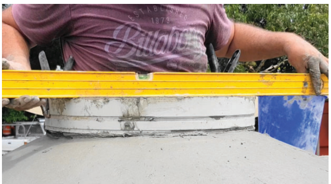
A thin sheet of plastic around the hob helps smooth it off, keep it circular and allow for taking a level
