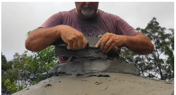
A thin sheet of plastic around the hob helps smooth it off, keep it circular and allow for taking a level
