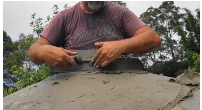
The ring is hand rendered with a trowel
