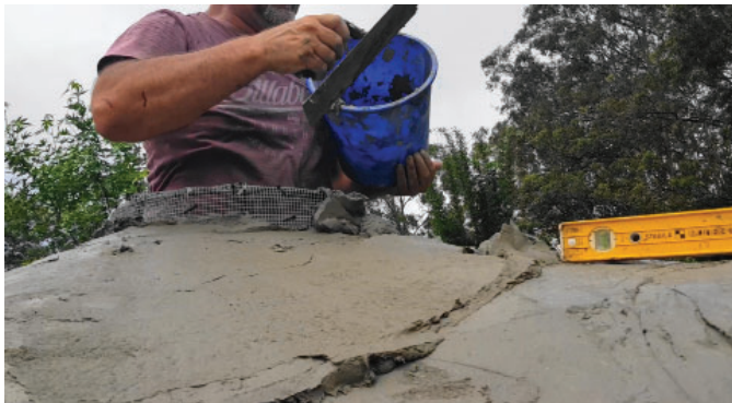
The ring is hand rendered with a trowel
