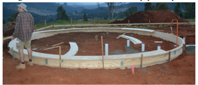
The formwork is fixed in place at the finished height of the slab - sewer and drain pipes in place
