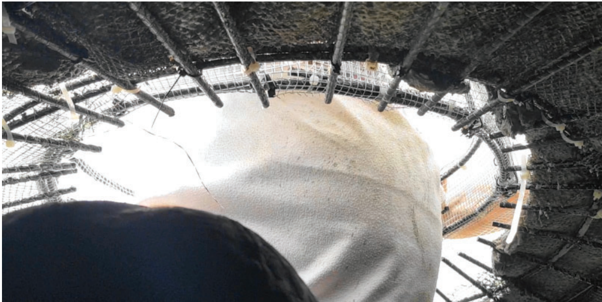
The ring is hand rendered with a trowel
